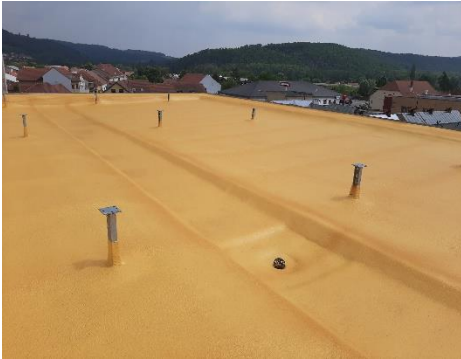
Roof after spraying PUR foam
