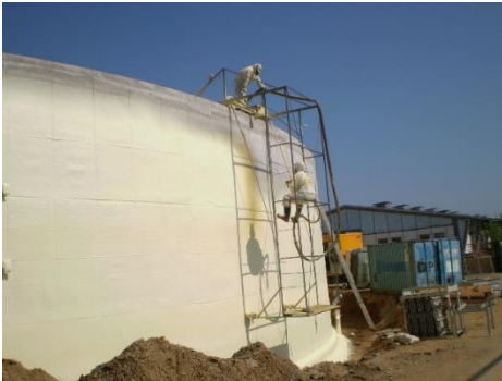
Thermal insulation of the exterior Fermenter shells
