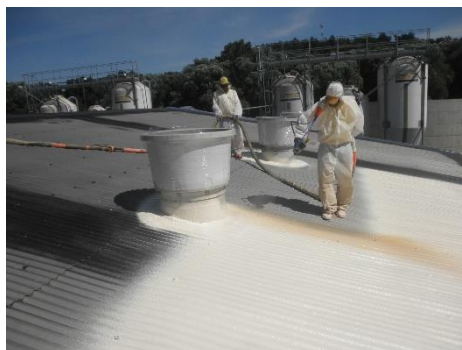
Spraying roof insulation animal production (aluminium sheet)
