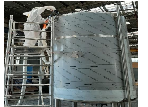
Tank insulation – PUR foam pouring "Filling holes"
