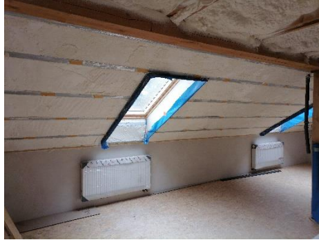
Spraying the attic on Contact diffusion layer
