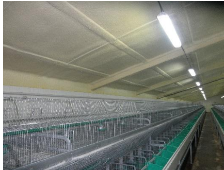
Insulation of the ceiling structure for rearing rabbits
