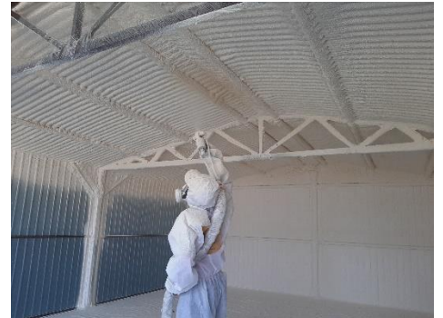
Insulation of a steel garage Anti-condensation
