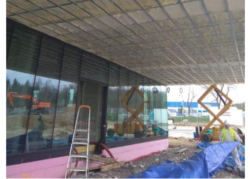
Insulation of ceilings concrete ceiling
