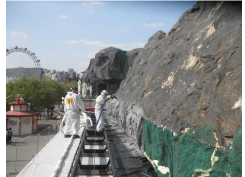
Spraying the decoration of the rock (Prater Amusement Park, Austria)
