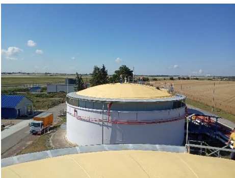
Application of insulation to storage tank (steel sheet)
