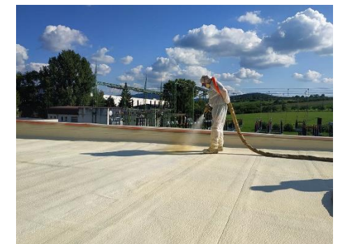
Spraying of industrial roof insulation Halls (asphalt strips)
