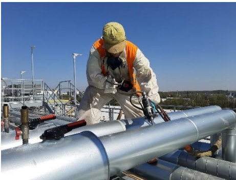
Pipe insulation - PUR casting foams "through filling holes"
